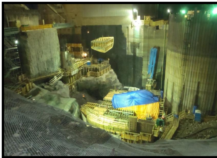
Figure 4: Kipling draft tube formwork module.
