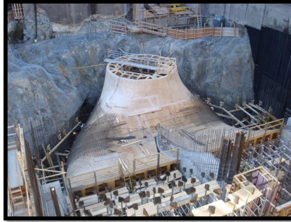
Figure 3: Curved wood forms for the draft tube at Little Long
