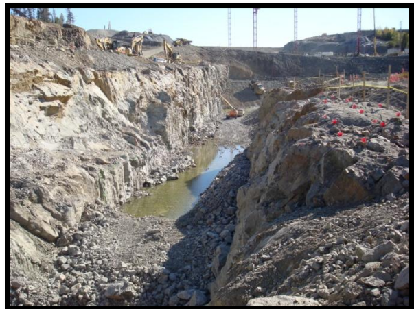
Figure 2: Excavation at the Smoky Falls Tailrace
