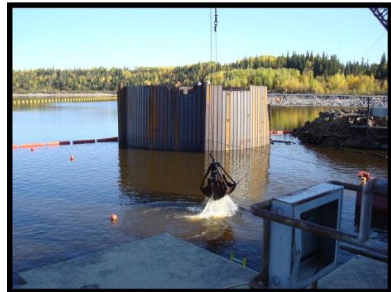
Figure 5: Cleaning the Footprint of Cell 2 and 3 at Kipling
