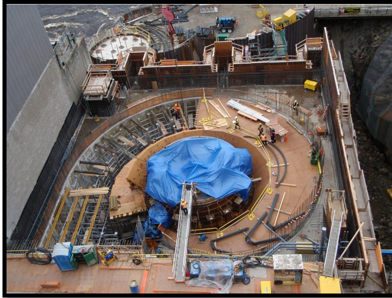
Figure 2: Harmon overview, scroll case soffit work
