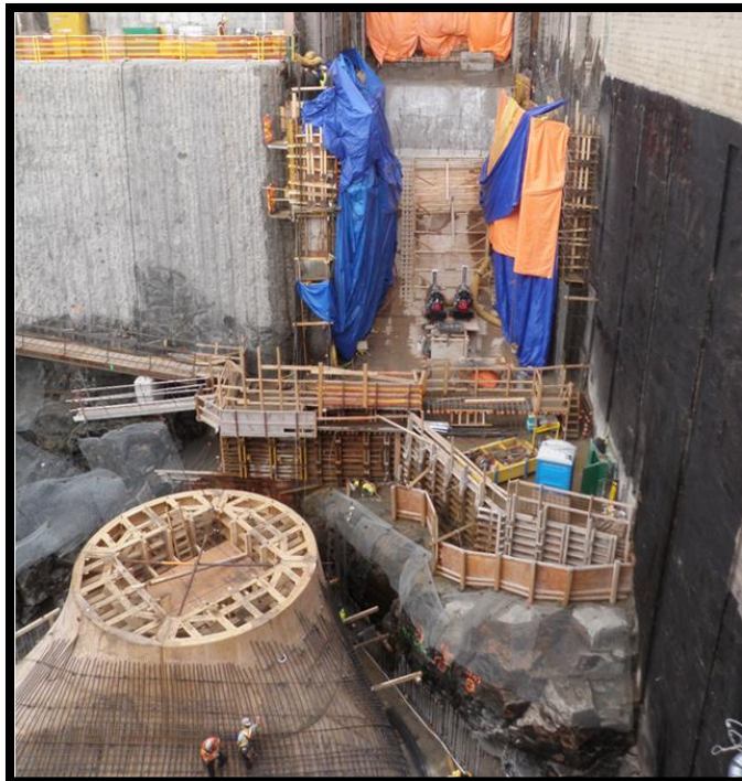
Figure 3: Kipling overview, intake and draft tube work.
