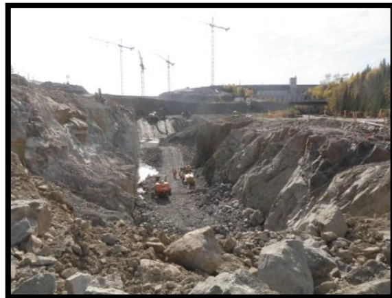
Figure 2: Excavation of Smoky Falls Tailrace
