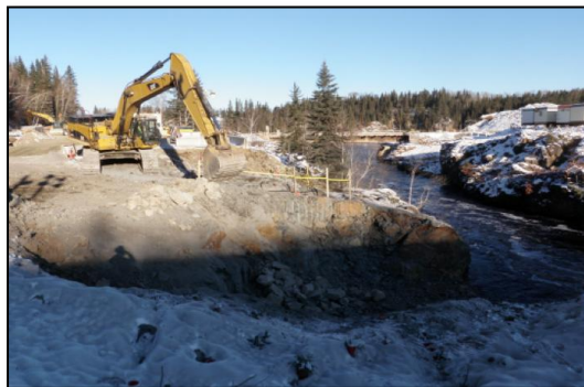
Figure 2: Smoky Falls – Excavating the West Permanent Bridge Abutment
