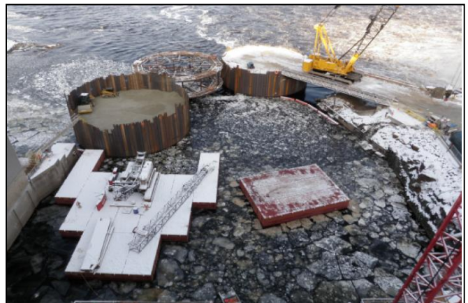
Figure 5: Kipling – Cofferdam Cell #2 Installation
