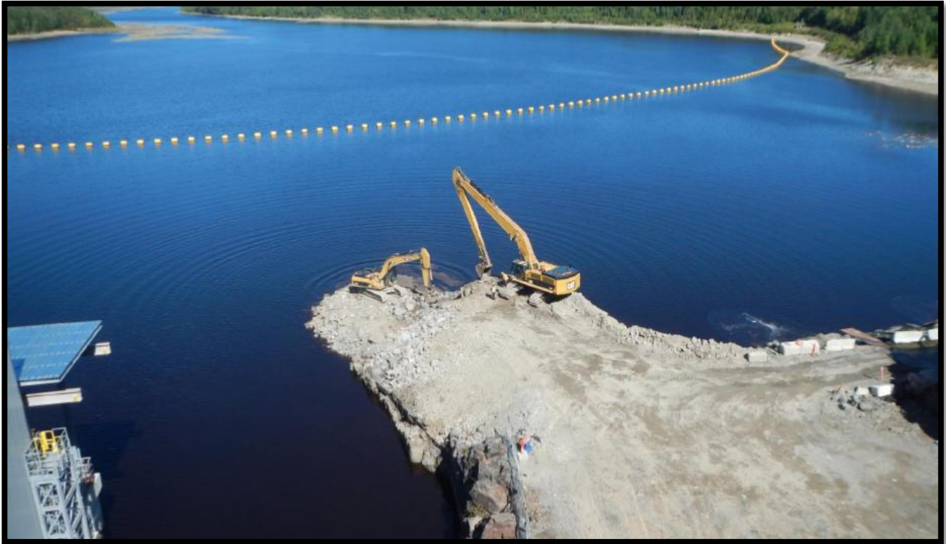
Figure 3: Kipling Cofferdam Backfill Operation
