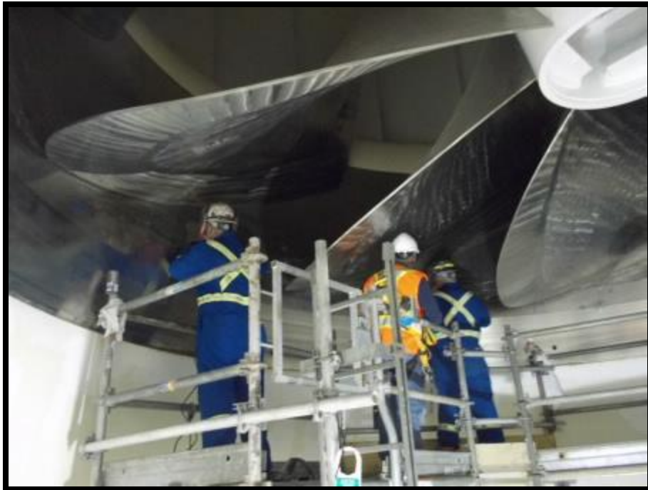
Figure 1: Little Long discharge ring grinding.
