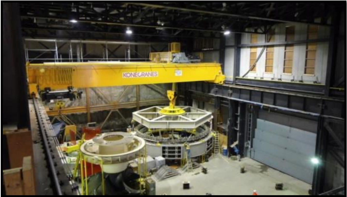
Figure 5: Smoky Falls: Unit 1 Stator Lift
