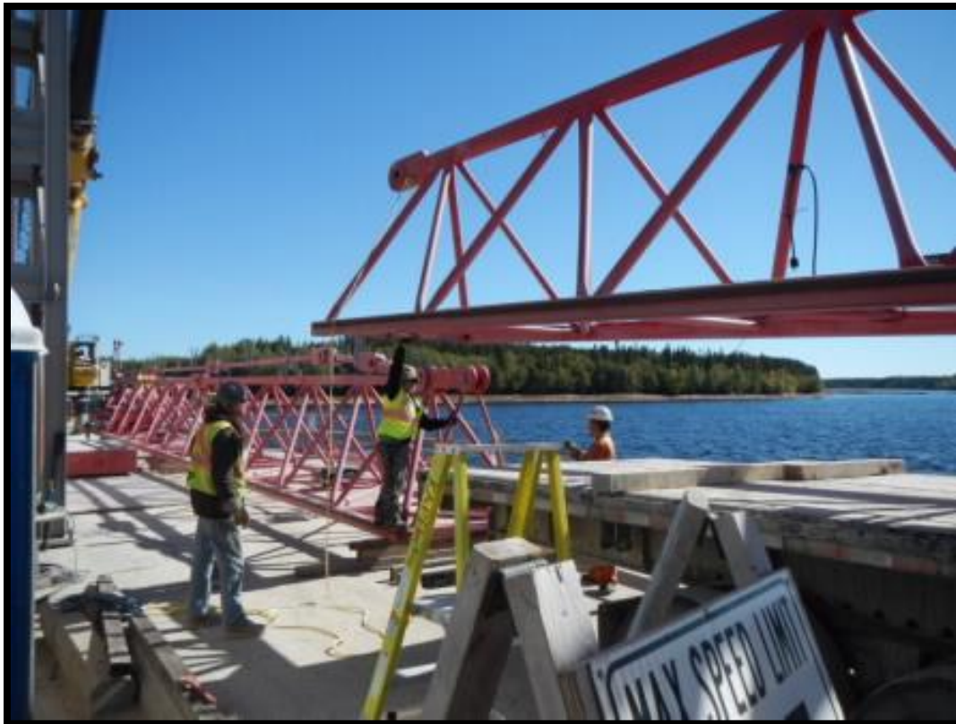
Figure 2: Harmon Cofferdam Template Removal
