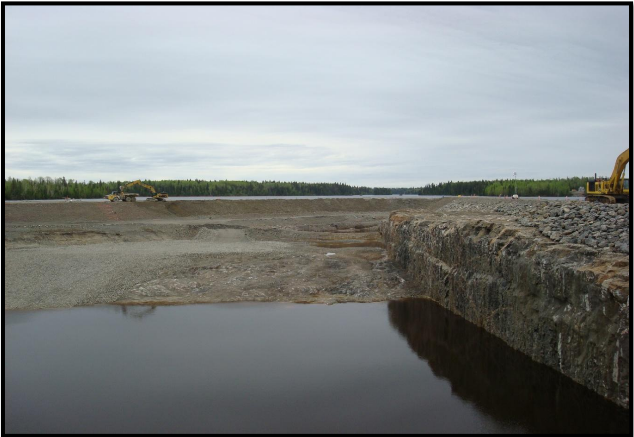
Figure 5: Smoky Falls cofferdam excavations
