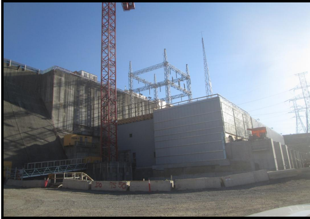
Figure 2: Kipling 230 kV switchyard towers erected
