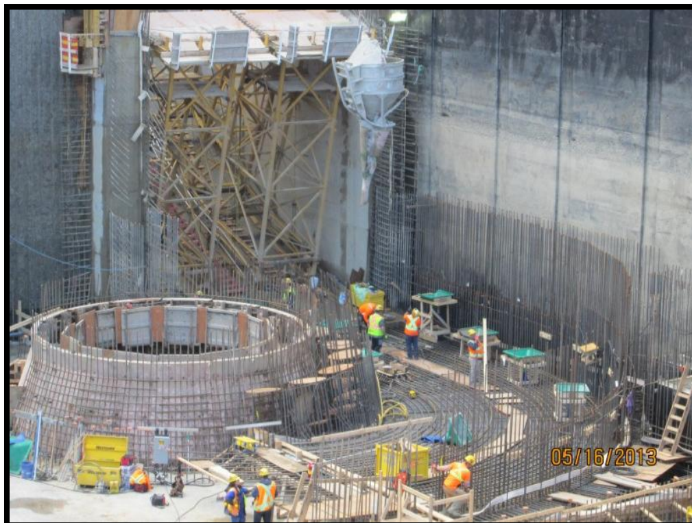
Figure 5: Concrete pouring at Kipling
