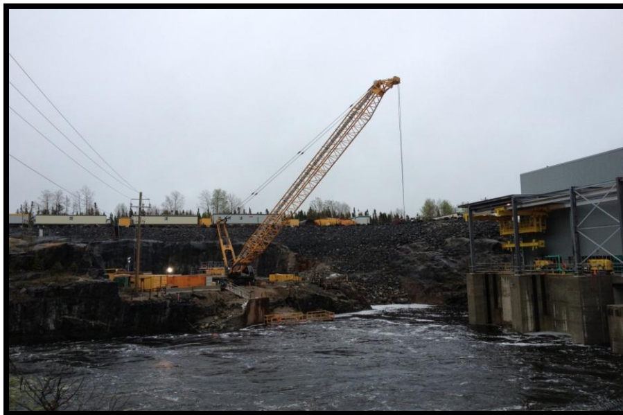
Figure 1: Little Long cofferdam removal
