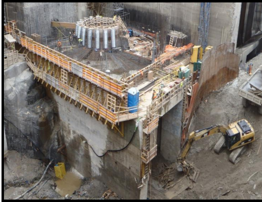
Figure 4: Sand Removal from Kipling Draft Tube
