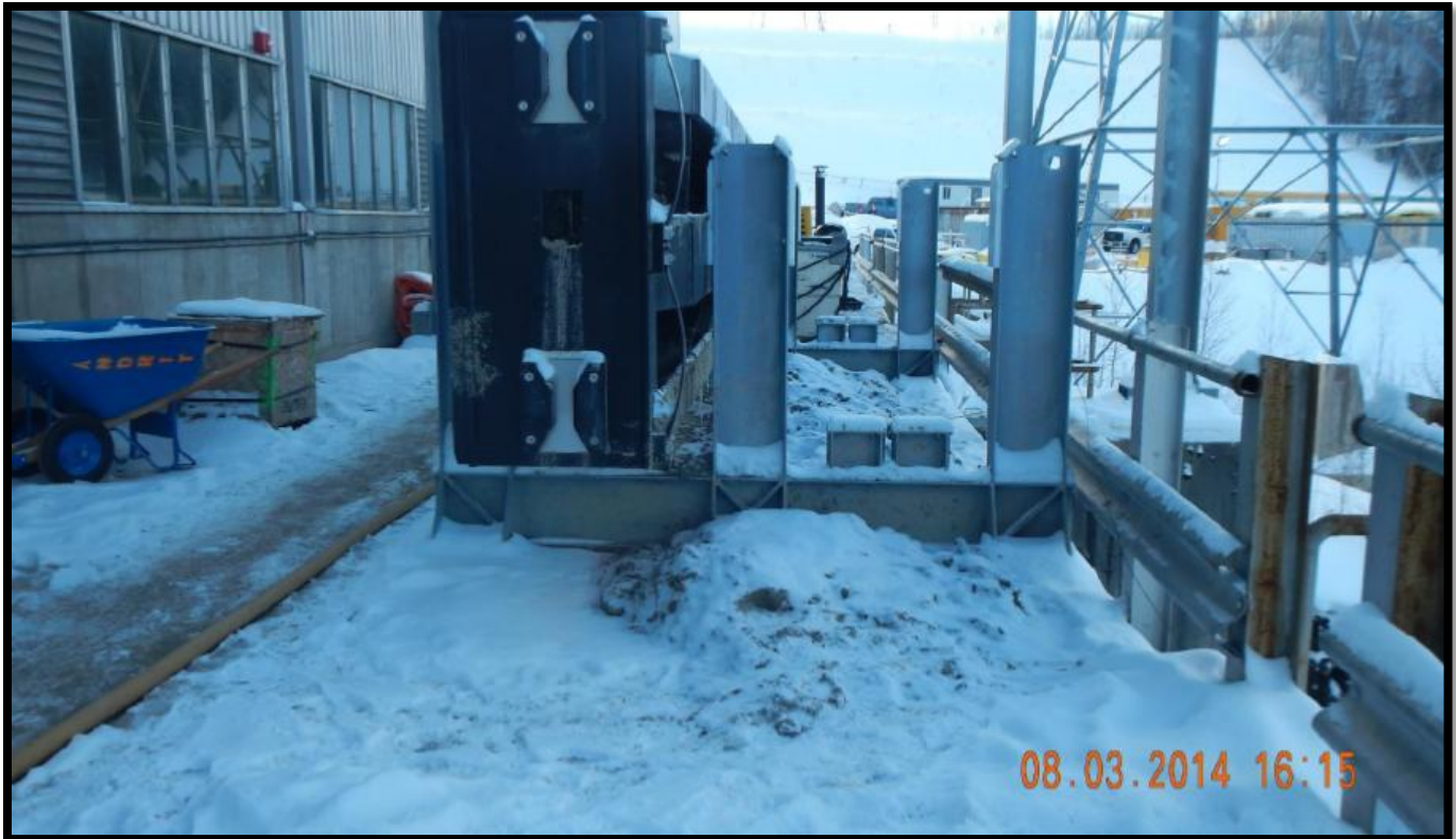
Figure 2: Harmon stop log and accumulated sediment
