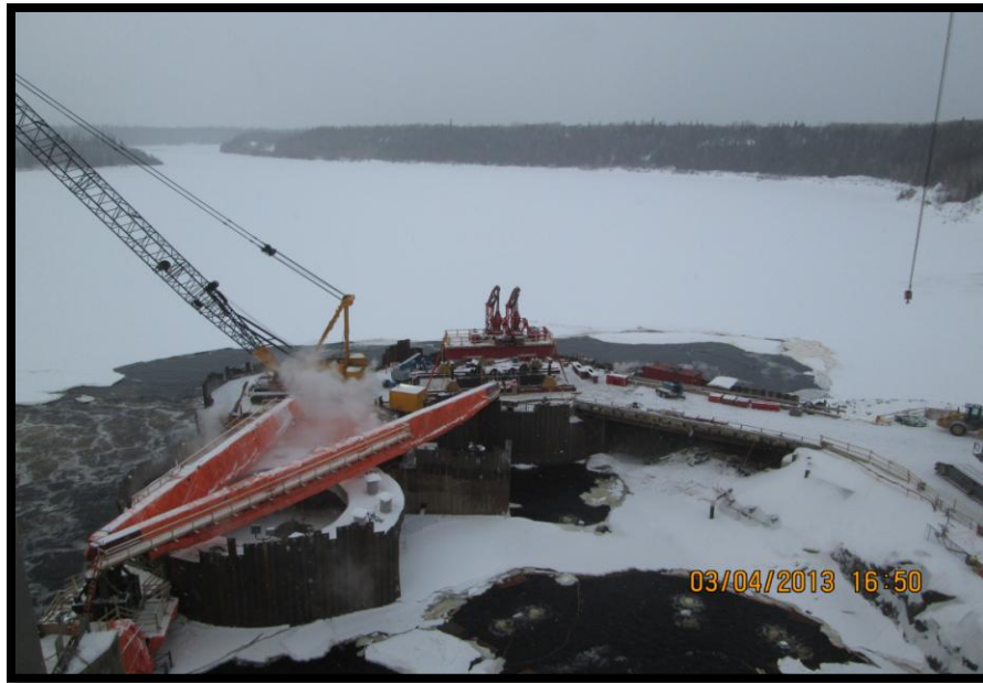
Figure 4: Kipling Jack Beam Assembly
