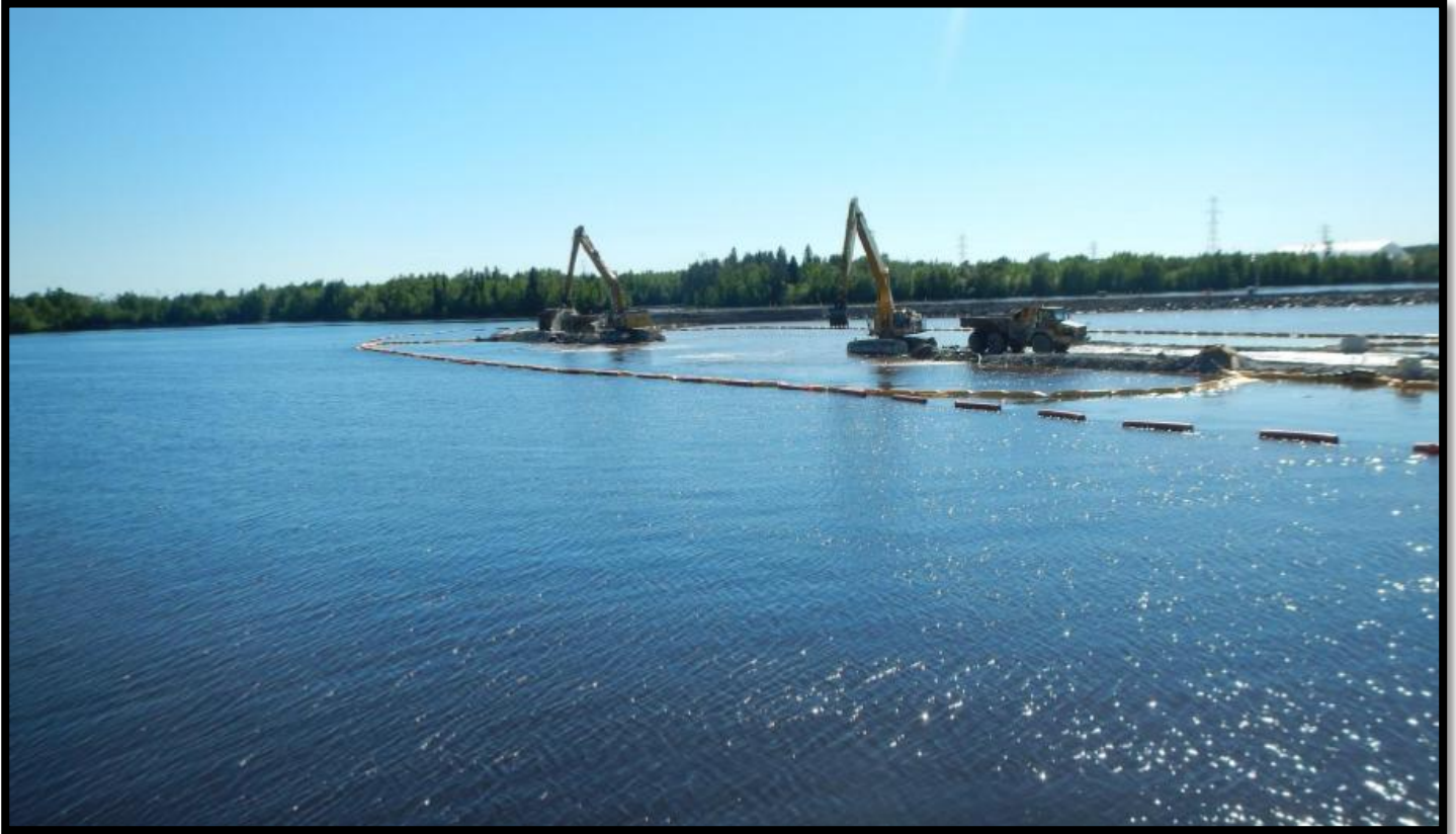
Figure 4: Smoky Falls cofferdam excavations
