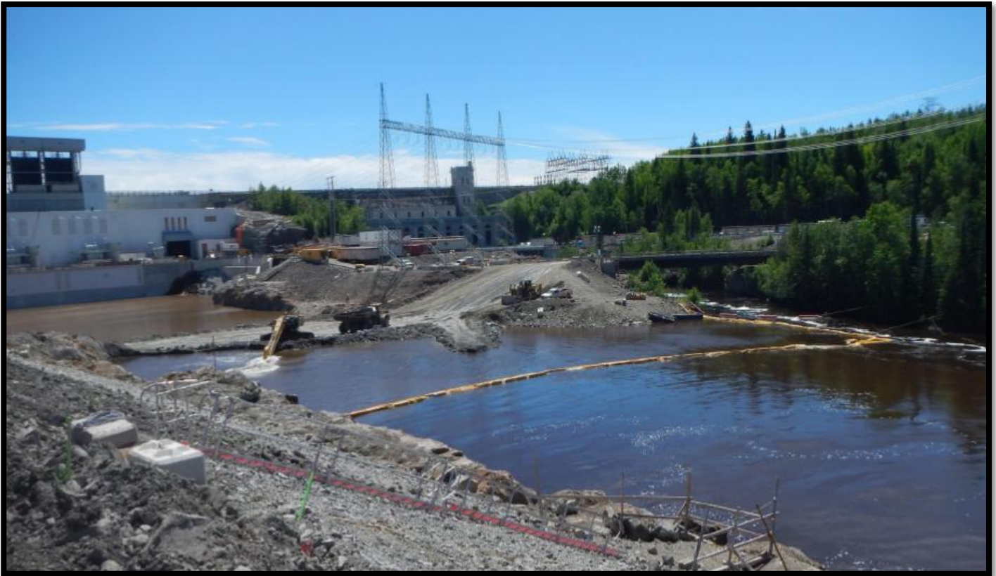
Figure 5: Smoky Falls rock plug excavations
