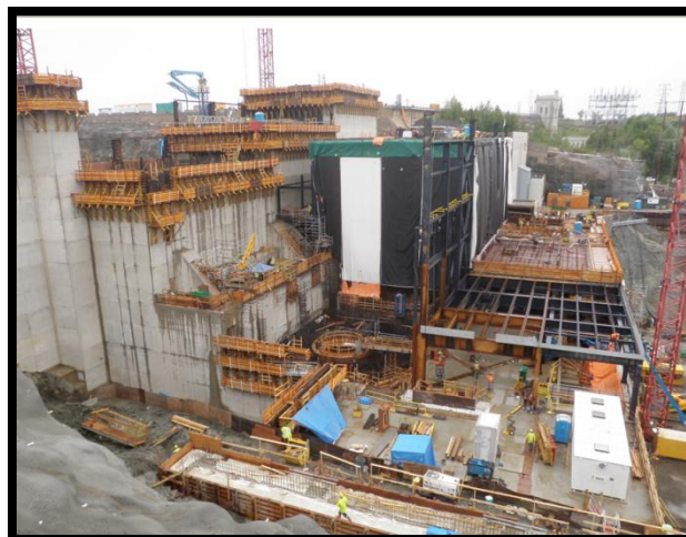
Figure 5: Smoky Falls: Overview of Unit 3 Superstructure Erection
