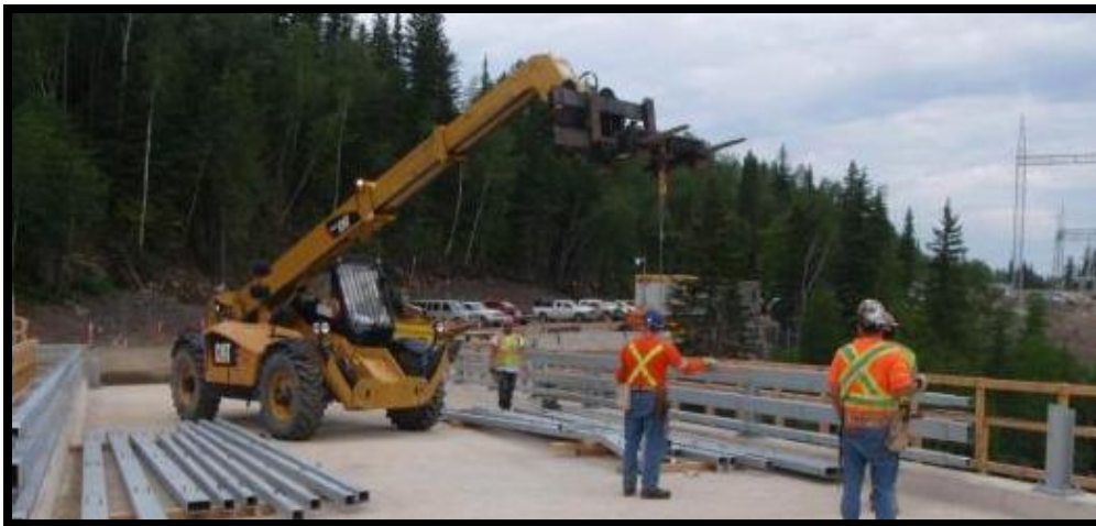
Figure 4: Smoky Falls: Installing guardrails at permanent bridge
