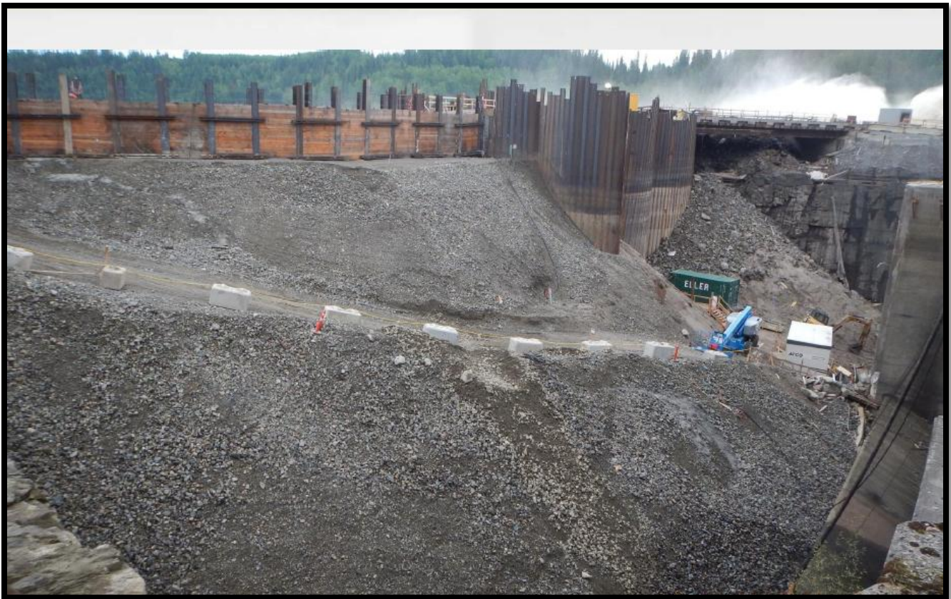
Figure 3: Kipling – Preparation work for removing fill material from the cofferdam earth berm
