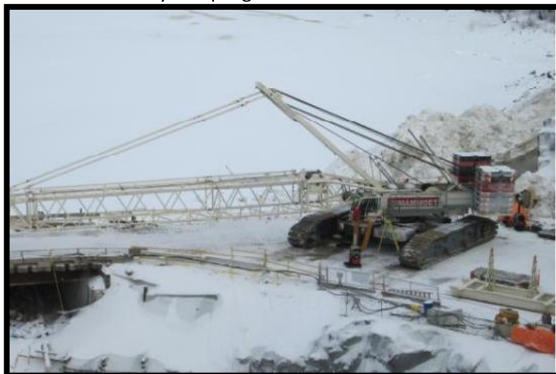
Figure 3: Mammoeth Crane Assembly
