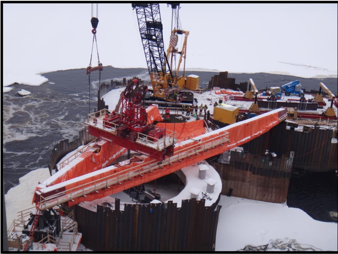
Figure 3: Troll Beams to stabilize the Cell 3 concrete ring
