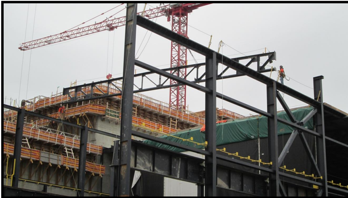
Figure 5: Smoky Falls: Unit 3 superstructure erection
