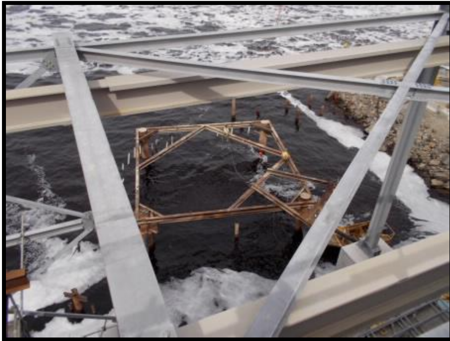
Figure 2: Harmon Cofferdam Template Removal
