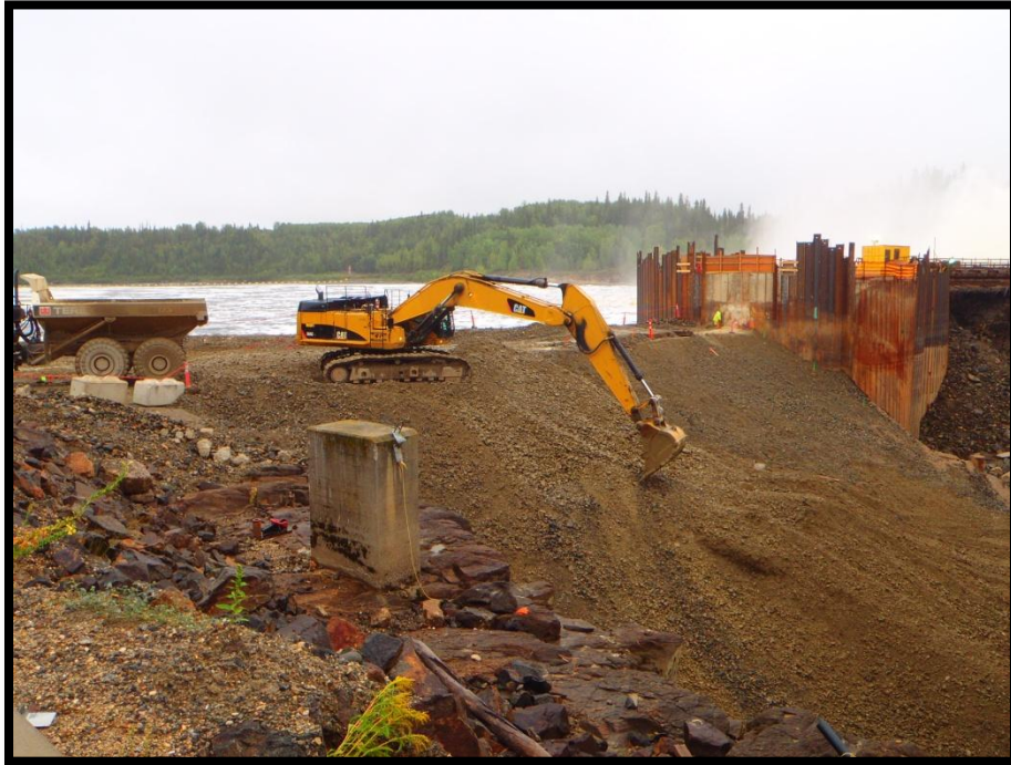
Figure 3: Kipling – Removing road from Kipling cofferdam
