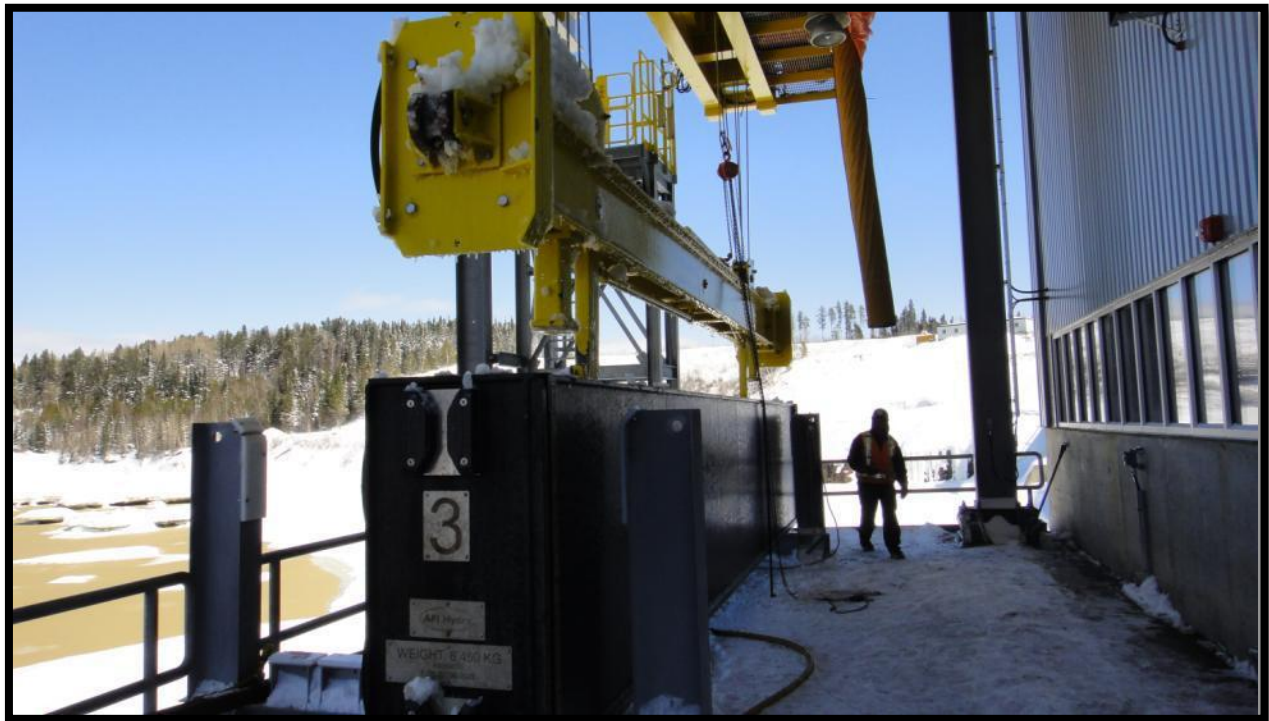
Figure 2: Harmon stop log removal
