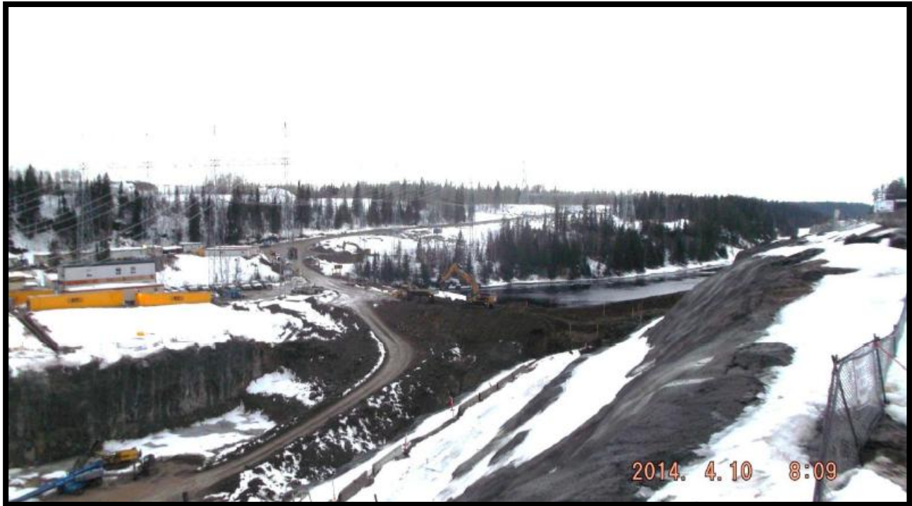
Figure 4: Smoky Falls – Rock-plug excavations
