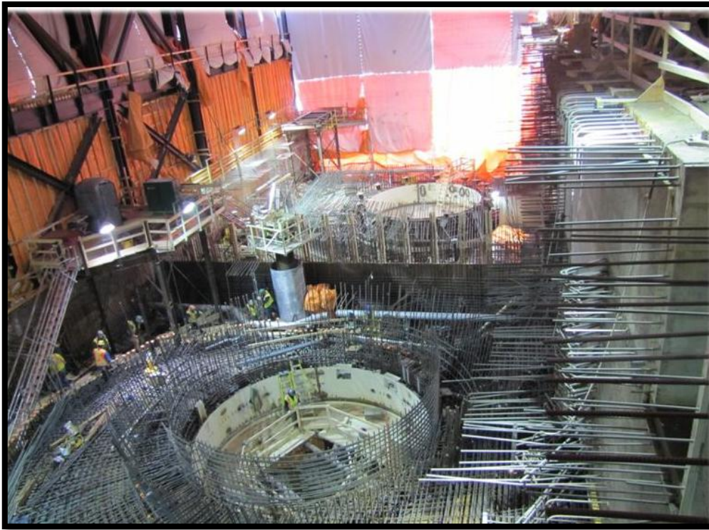
Figure 3: Smoky Falls Unit 1 and 2 Scroll Case
