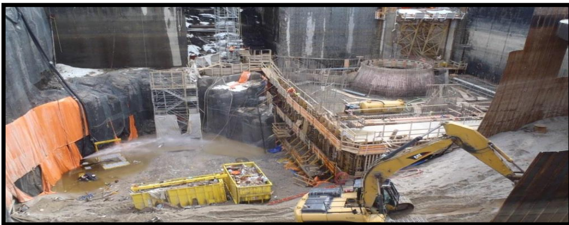
Figure 5: Kipling debris clean-up within dewatered lagoon
