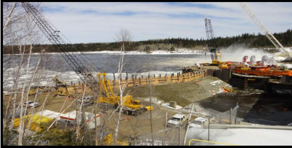
Figure 4: Kipling Completed Lagging Wall (with H-piles and sheet piles)
