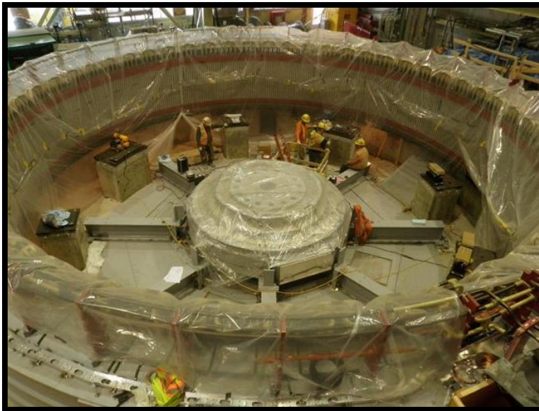
Figure 1: Little Long assembling the lower brackets
