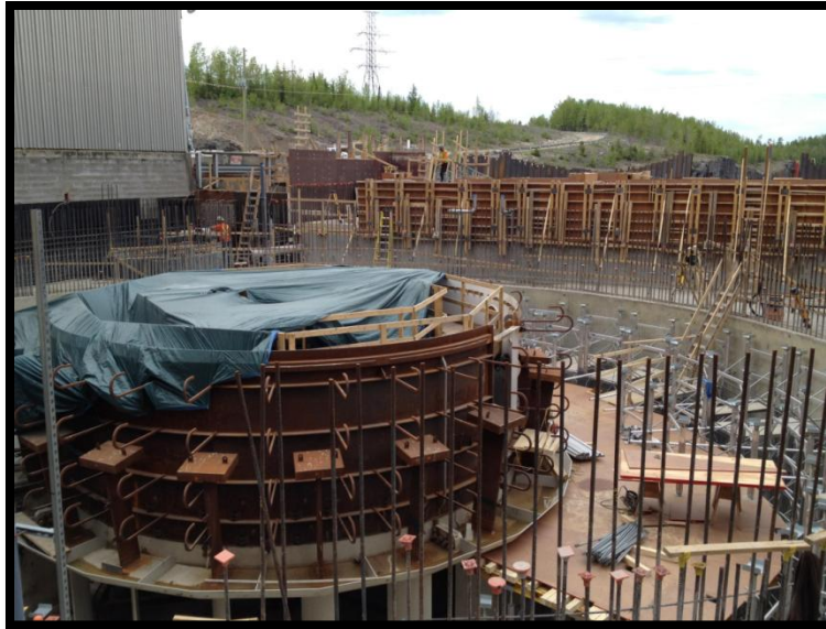
Figure 1: Little Long Pit liner, scroll case shoring and stay ring
