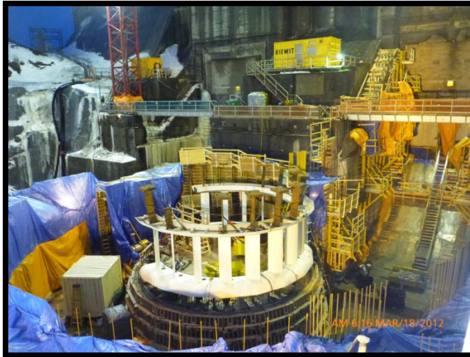
Figure 1: Formwork and stay ring at install at Little Long Powerhouse
