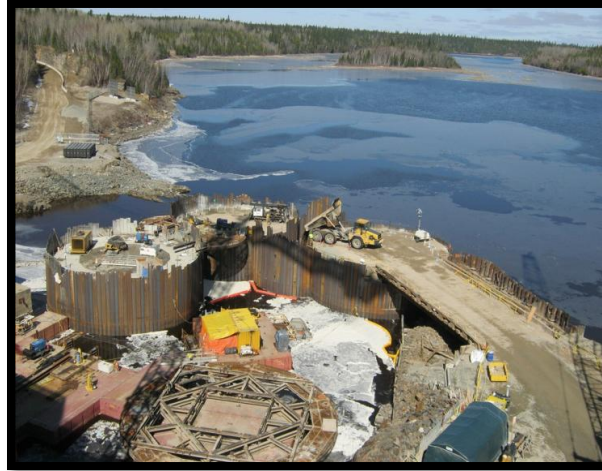
Figure 3: Sand Backfill at the Kipling cofferdam
