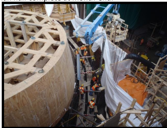
Figure 4: Draft tube pour at Smoky falls
