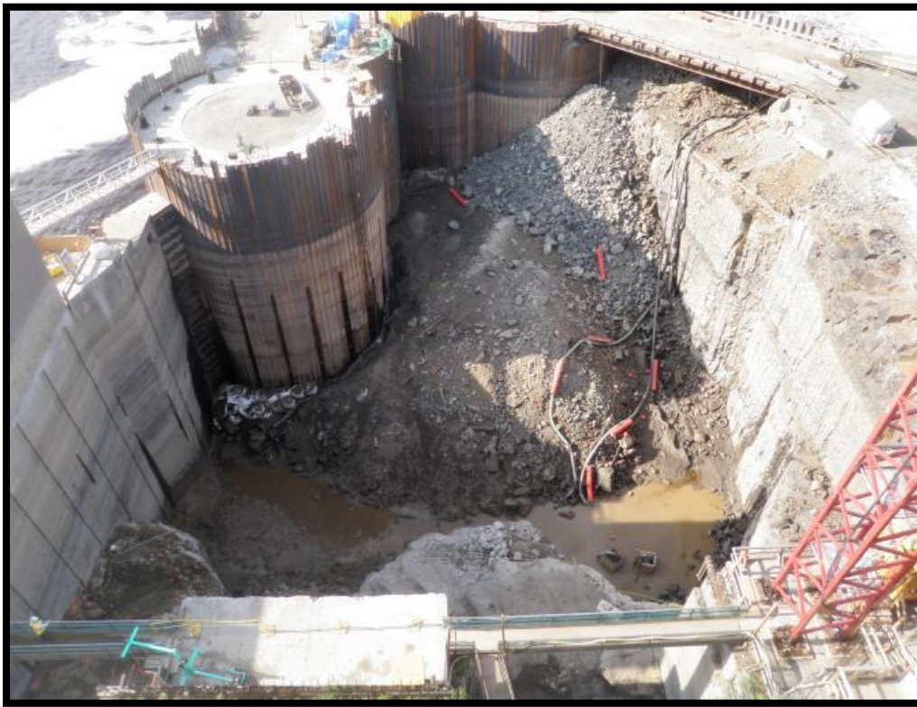
Figure 3: Kipling dewatering completed on June 25
