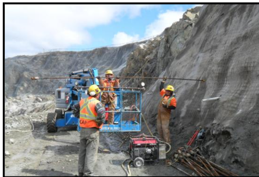
Figure 2: Installing the rockbolts on the East Wall in Zone 1
