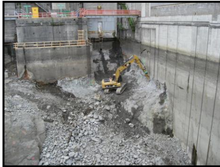
Figure 3: Excavation operation in the Bull Nose area
