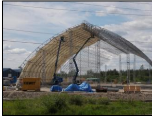
Figure 1: Megadome - Installing the first tarp
