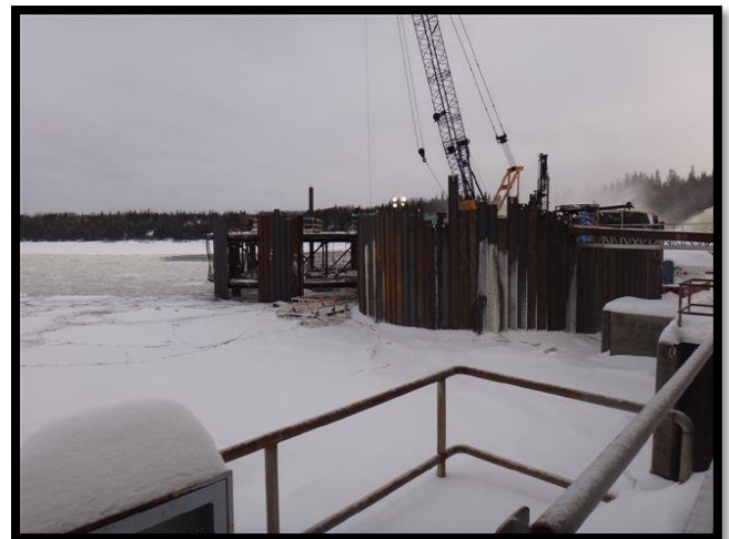
Figure 5: Kipling – Installing Cell #2 Sheet Piles
