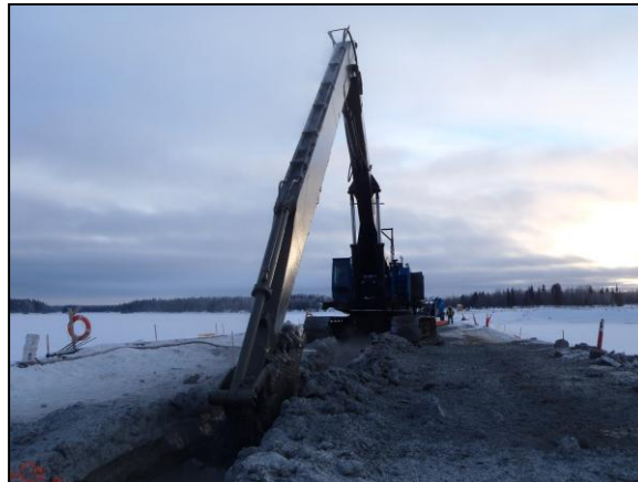
Figure 1: Smokey Falls Cut-off at the Cofferdam
