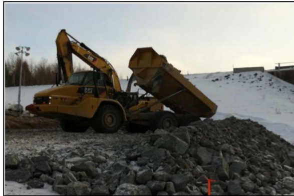
Figure 3: Dumping blast rock at Harmon
