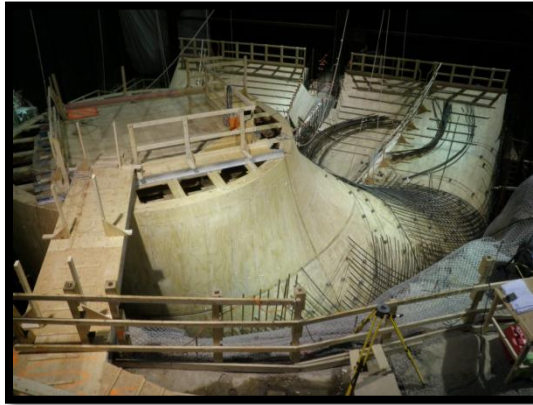
Figure 3: Draft tube work at Harmon
