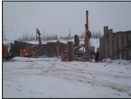
Figure 3: Grout drilling operation on top of the Little Long cofferdam.
