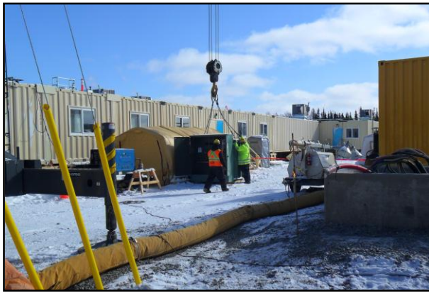
Figure 1: Placing the containment pit at the Smoky Falls Permanent Camp
