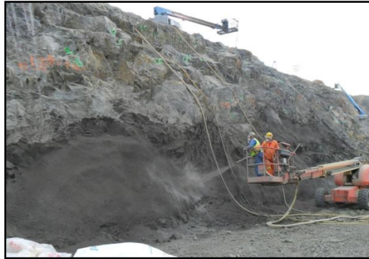
Figure 1: Applying shotcrete in Zone 3
