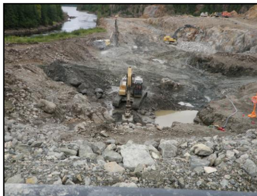
Figure 2: Smoky Falls Wet Tailrace Excavation
