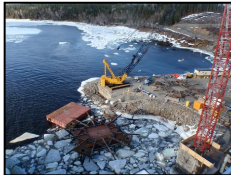
Figure 4: Working on the template assembly at Harmon
