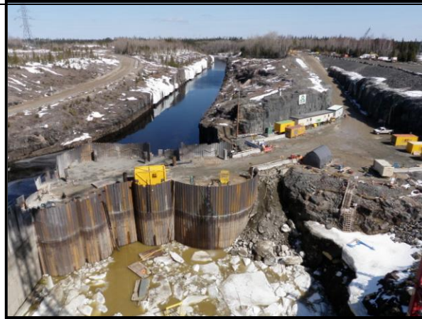
Figure 3: Dewatering at Little Long cofferdam
