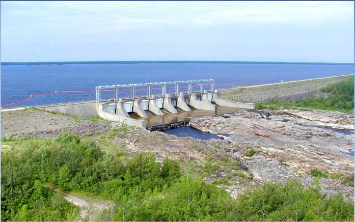
8 spillway gates that each have the capacity to pass 600cms each. Total spill capacity of 4870cms (1.3 million gallons per second or 111 billion gallons per day). Average spring spill at Adam Creek 1250cms (330,215 gps or 28.5 billion gpd).
